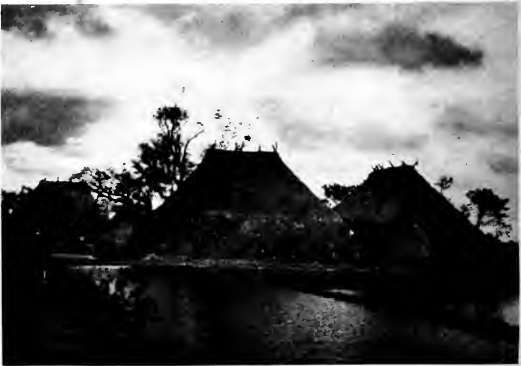
Ice reaches its farthest south in Ningpo, where it is "grown" on shallow ponds and stored away, no thicker than window-glass, in ice-houses of earth and thatch
